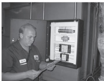
Jim Koehler, HVAC Technician
