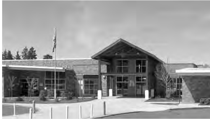
Jason Lee Middle School: When the AC system failed, it triggered a series of changes because excessive cost of repairs necessitated a better solution. The mechanical maintenance team decided to install a new air-cooled chiller with high efficiency compressor, to replace the electric heating system boiler with high efficiency equipment and to update the kitchen walk-in cooler and freezer. The annual net savings for this project are calculated at just over $50,000.
