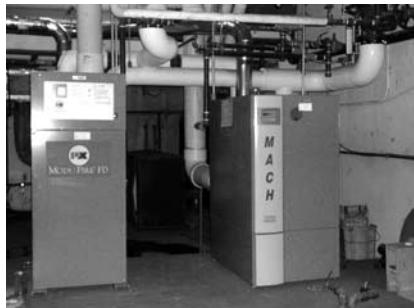
Modulating boilers replaced a broken system, saving an estimated $7,200/year in heating costs.
