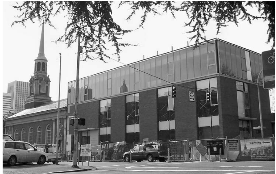
Construction in progress on the First Unitarian Church of Portland's LEED-certified building.
