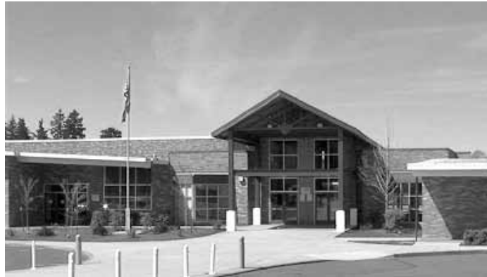
Jason Lee Middle School: When the AC system failed, it triggered a series of changes because excessive cost of repairs necessitated a better solution. The mechanical maintenance team decided to install a new air-cooled chiller with high efficiency compressor, to replace the electric heating system boiler with high efficiency equipment and to update the kitchen walk-in cooler and freezer. The annual net savings for this project are calculated at just over $50,000.
