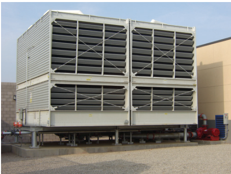
Cooling tower at FHS that allows chillers to run more efficiently than in an air-cooled system.
