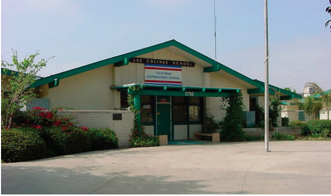
Los Colinas Middle School in Pleasant Valley School District.
