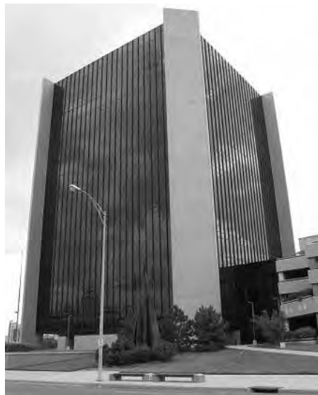
Wichita City Hall: a 350,000 sq. ft. building that is the center of city facilities monitoring.
