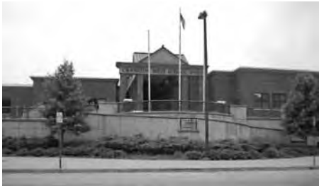
Cranston West High School, one of twelve schools to receive the EnergyStar® label in the district.
