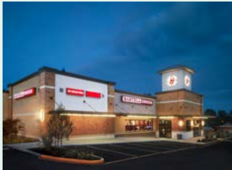
Bartell Drugs' Lynnwood, Washington location has 25-watt T8 linear fluorescent lamps installed to save energy and money.
